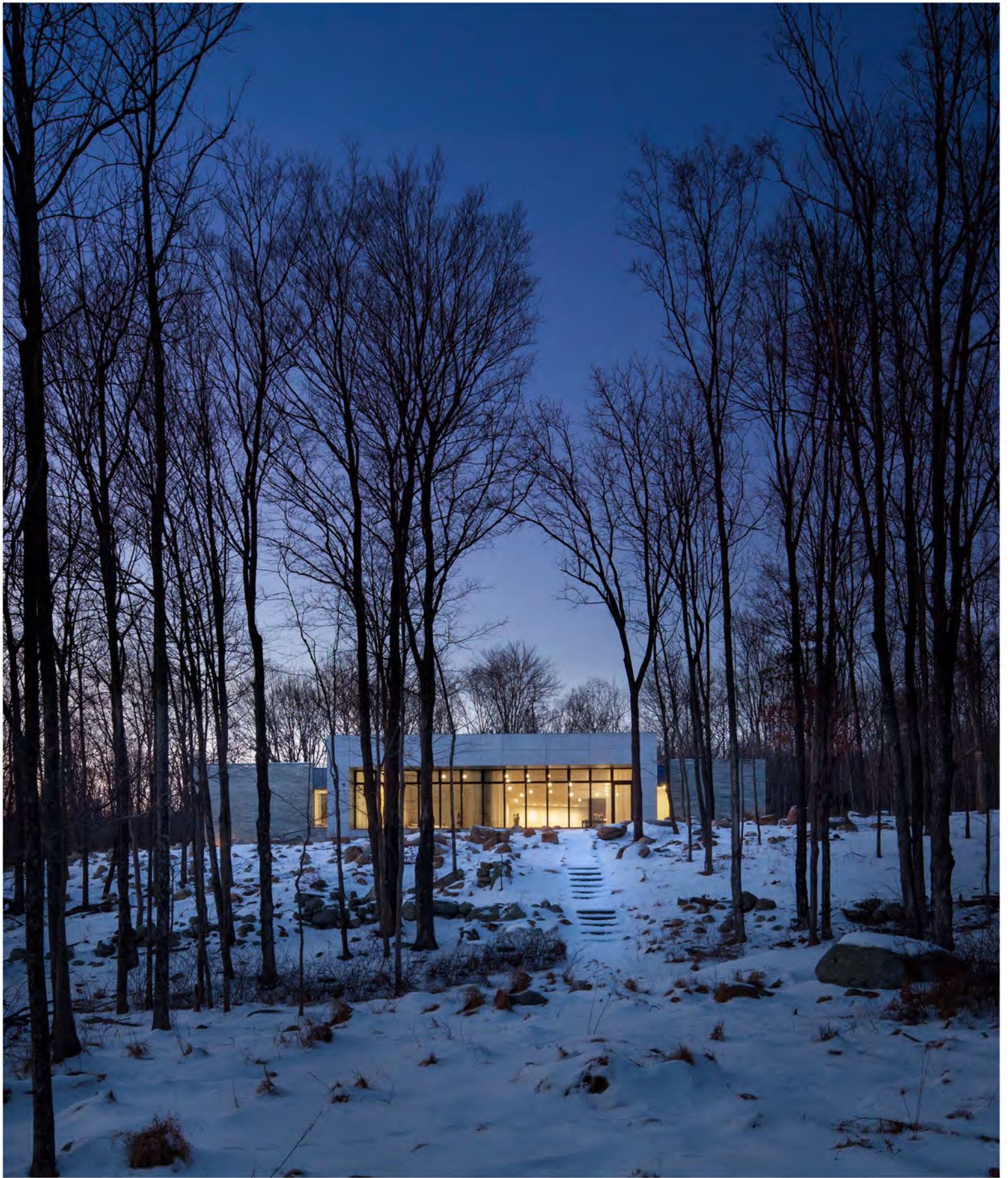
— The rear elevation of A House in the Woods appears to hover slightly above the forested hillside.
